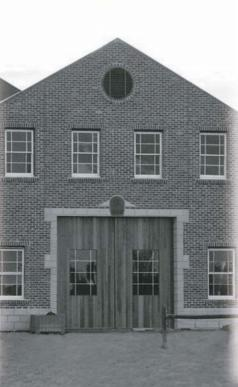
some reclaimed materials, such as the double hung casement windows from a 1930s hospital, old leadlight windows and doors, plus large plinth and door reveal stones. Several aspects of the building are state of the art, such as the cast in Taylors stainless steel drains from New Zealand, and some are leading edge technology, such as the Bonacci Beams (designed by leading structural engineer and friend, Nat Bonacci) – this was the first use of this revolutionary patented building system.
